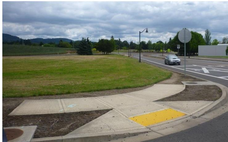
ADA Compliant Curb Ramp with No Connections
